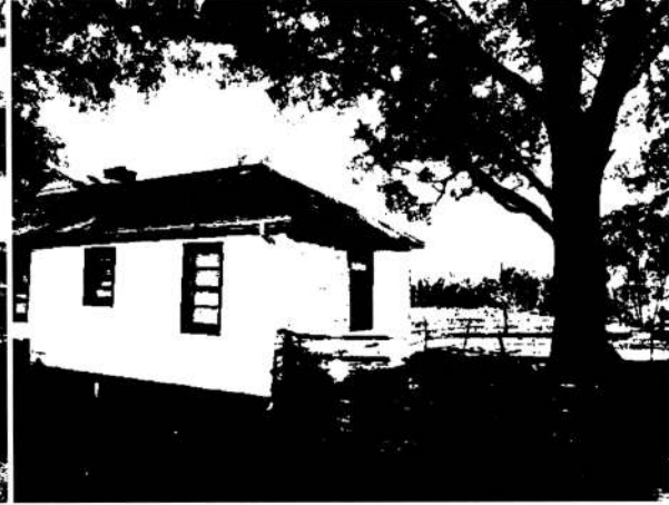
26. Back portion of the house.
