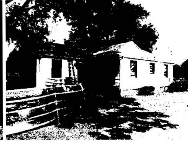
28. South side of the house.
