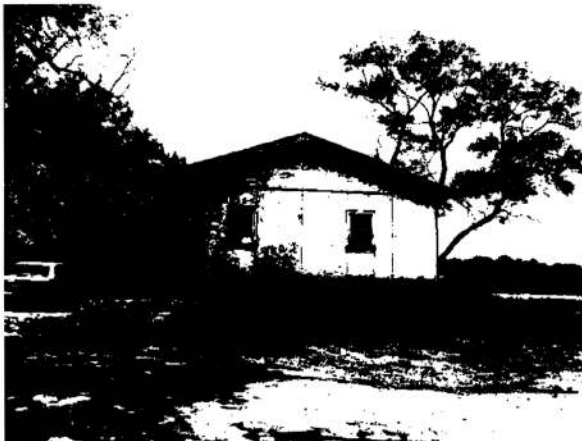
23. House being removed from the 4-acre parcel.
