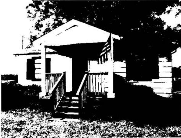
25. House used for the construction office. Front view.
